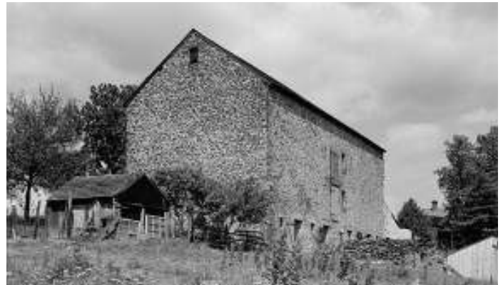
Stone barn in Newtown, Bucks Co. (Courtesy HABS #PA 5332-1)
