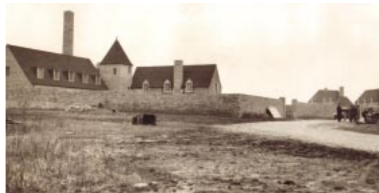
Figure 6 (below, bottom) Staff cottages under construction, Newtown, Pennsylvania. Undated photograph, ca. 1930.
